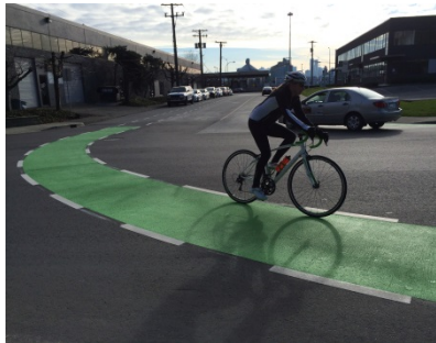
Welch Street (completed 2014) On-street bike lanes to connect the Spirit Trail to 1st Avenue on-street bike lanes.
