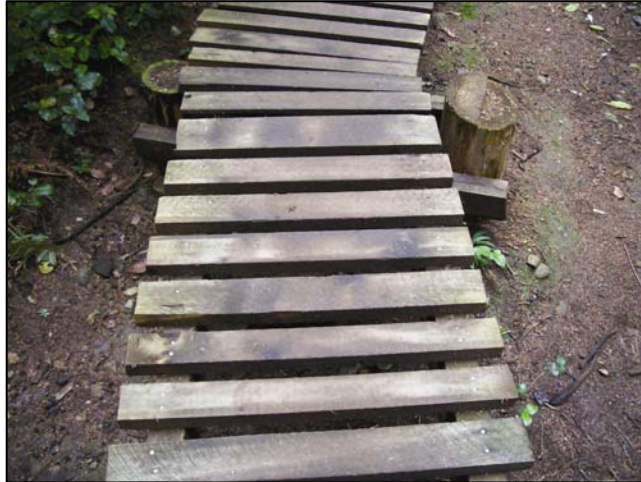
Two inch bridge rung spacing prevents foot and paws from falling through while allowing dirt to shed from the structure, Natural High, Fromme Mountain.
