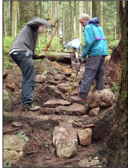
Figure 17: Protecting tree roots with rock armouring.
