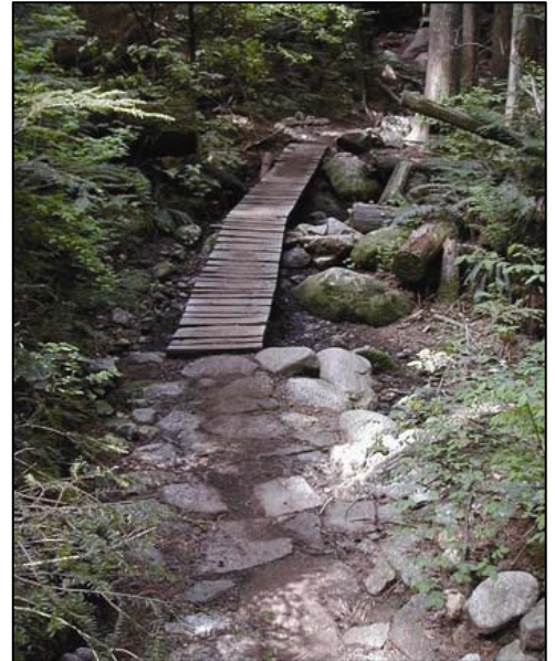
Figure 2: Incorporating bridges near surface drainage areas can mitigate the effects of diverted surface water flow.
